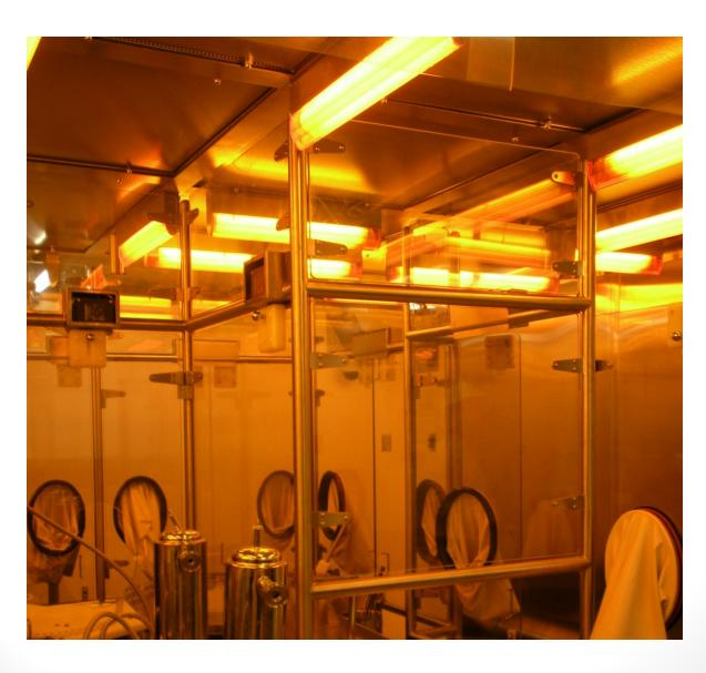
Typical fare is 304/316L SS FFU with a gel seal HEPA filter, fan status reporting, test ports, networked fan control, and a master system display
